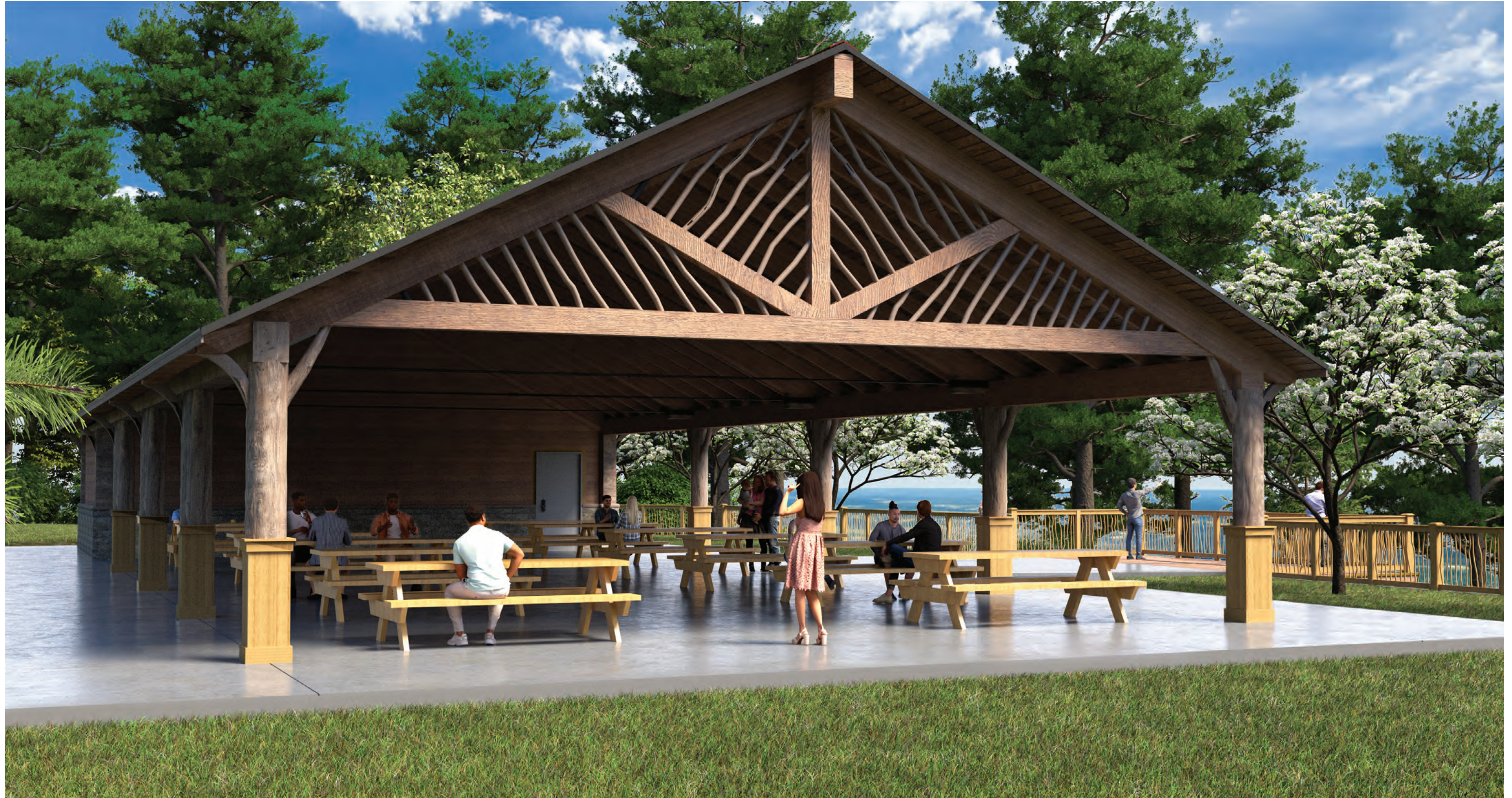
Above Image: Perspective rendering of the southern end of the Event Pavilion, highlighting the natural, wood branch infill of the roof truss and the Adirondack-style log-wrapped structural columns.
